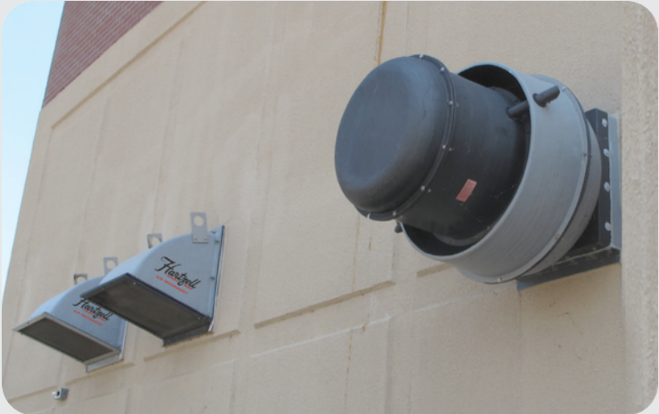
Series 88 Fiberglass Exhauster with Electrostatic Grounding and Hoods
