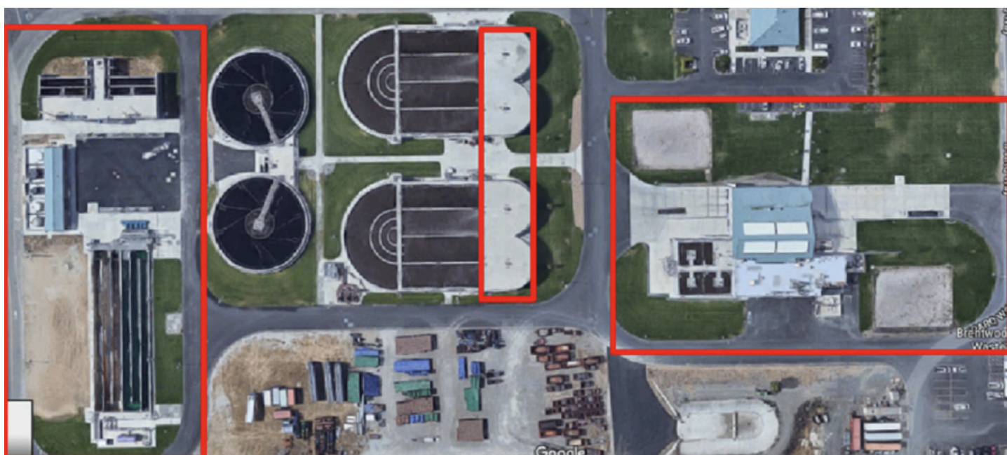
Wastewater plant installation with 30 fiberglass fans
