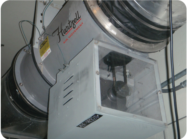
Series 35V Fiberglass Duct Vaneaxial Fan
